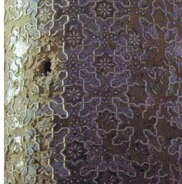
Figure 5: An existing pattern on the wall of Mossalâ , Herât, Afghanistan.
